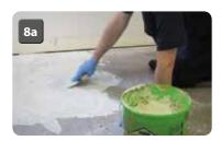
Starting with a few square meters at a time apply Mapei Ultrabond ECO 380 to the substrate using a 2mm (A2) tooth comb spreader (8a). Do not use Mapei Ultrabond ECO 380 as a filler to level out gaps, cracks or uneven substrates as this will greatly reduce the coverage achieved and increase drying times. Any uneven screed or concrete floors should be levelled with a renovation screed first.
