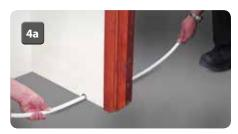
4. When floor heating pipes need to pass through walls, drill the holes before laying and fixing boards to prevent any damage to the boards. Protect and seal the pipe ends with tape. To prevent kinking, one person should feed the pipe through the hole whilst another draws the pipe through from the other side (4a).
