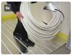
This will help deter the pipe from trying to twist, ease the pipe around and into the bend. Lay the pipe into the return or corner gently forming and pushing the pipe gently into the channel as it forms around the bend (9d/e).
