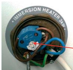
Check electrical connections & sensor are fixed properly and the overheat thermostat is set to 70C.
