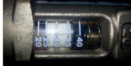
**If the flow rate is too low you need to fix this before moving on.**
