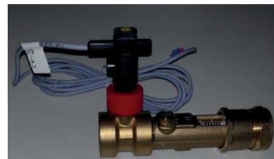
If you manually open the hot water 2 way valve check the flow rate again, if you can only reach 16l with the heating and hot water open together it's a sure sign the pump you have installed is too small.
