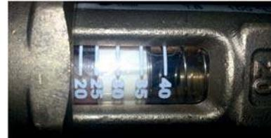
The flow switch trips out at 15l/min, if the flow drops below this E911 shows.
