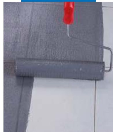
Application of Eco Prim Grip by roller on existing porcelain tiles
