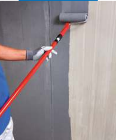
Application of Eco Prim Grip on concrete by roller
