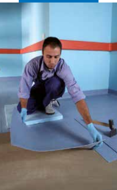
Installing PVC floor tiles
