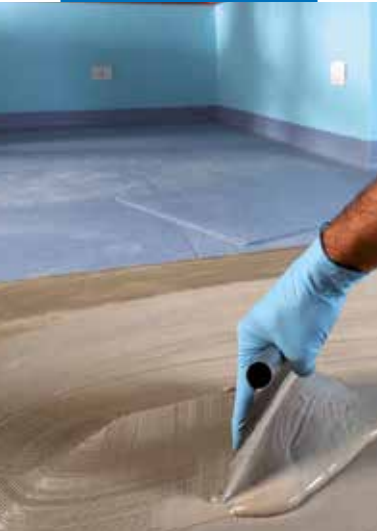
Applying Ultrabond Eco 380
